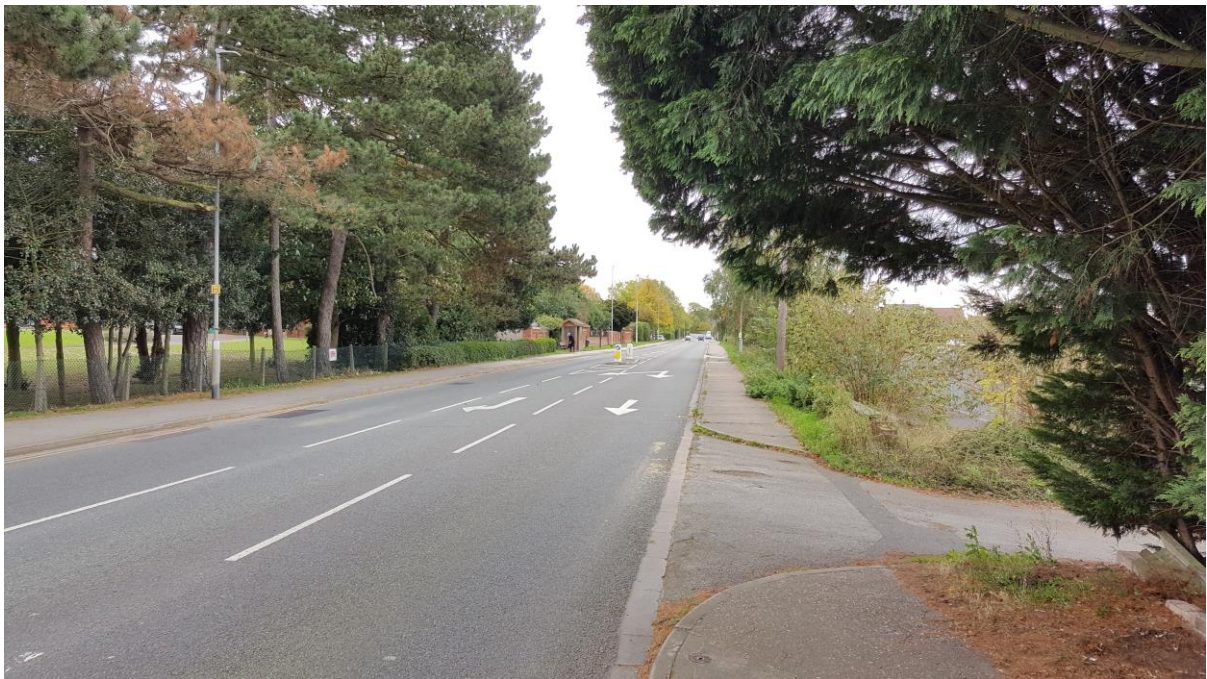
View South East Along Site Frontage (right of picture) with Long Leys Road (existing access to site visible)
