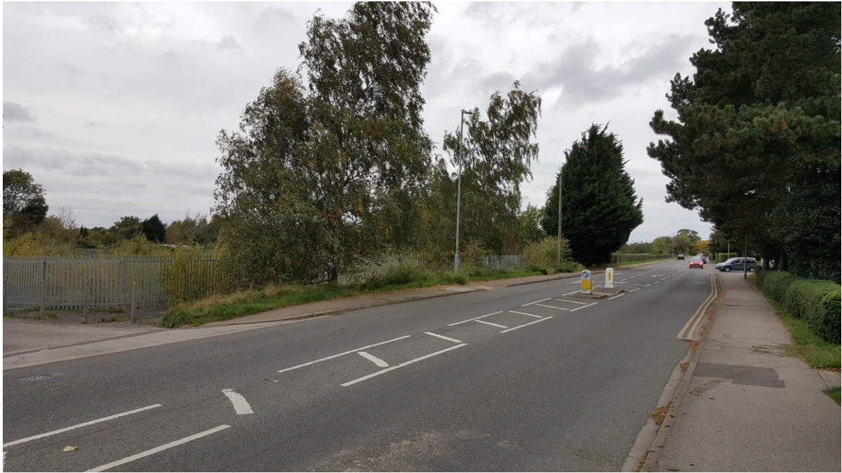
View North West Along Site Frontage (left of picture) with Long Leys Road
