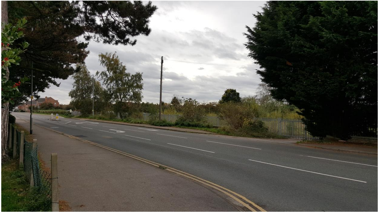
View South West Towards the Site Across Long Leys Road (Access to Site Visible)
